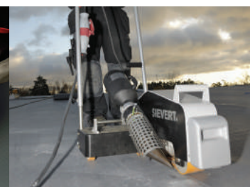
TW 5000 hot-air welding
